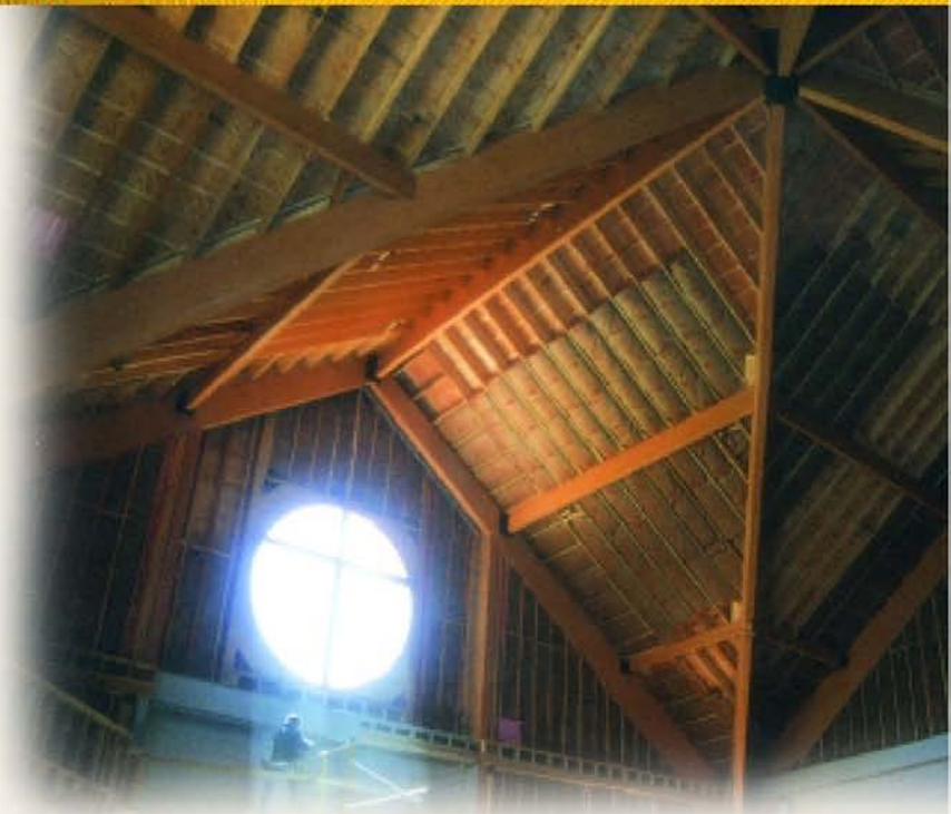
Rosedale Baptist, Sanctuary construction above
